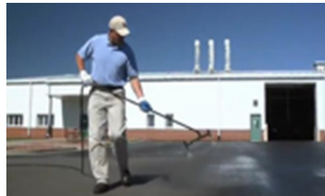
Figure 13. Application of RePlay (a) with a sprayer with a tank of RePlay loaded on the back of a pickup truck (BPS 2014) and (b) with a hand-held sprayer connected to a RePlay tank source.
