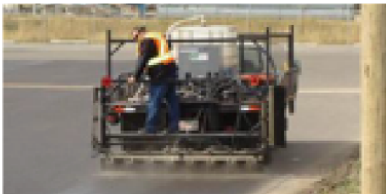
Figure 13. Application of RePlay (a) with a sprayer with a tank of RePlay loaded on the back of a pickup truck (BPS 2014) and (b) with a hand-held sprayer connected to a RePlay tank source.
